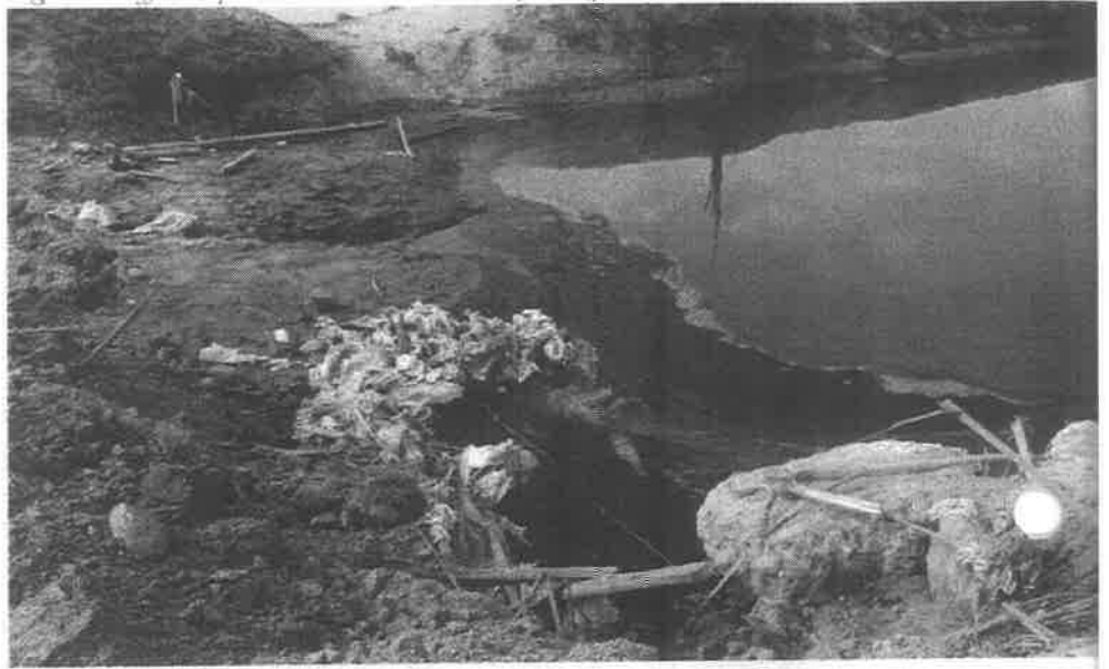
Figure 4. Effluent pits near BGN#5 with oily sludge and construction debris
